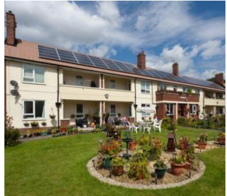
PV array on Stockport Housing Association
